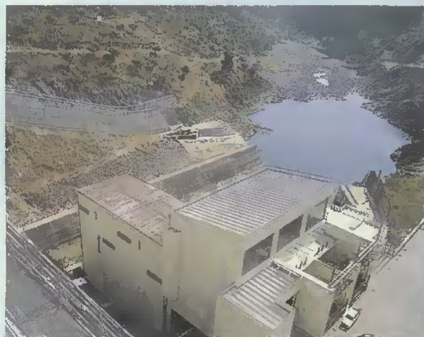
Central / Power Station
